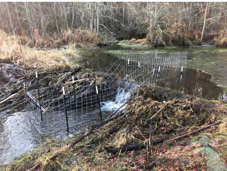
Figure 31: Example of a notch exclusion fence in Washington that allows for fish passage while still maintaining the desired water level behind the dam. Photo Credit: Beavers Northwest.
