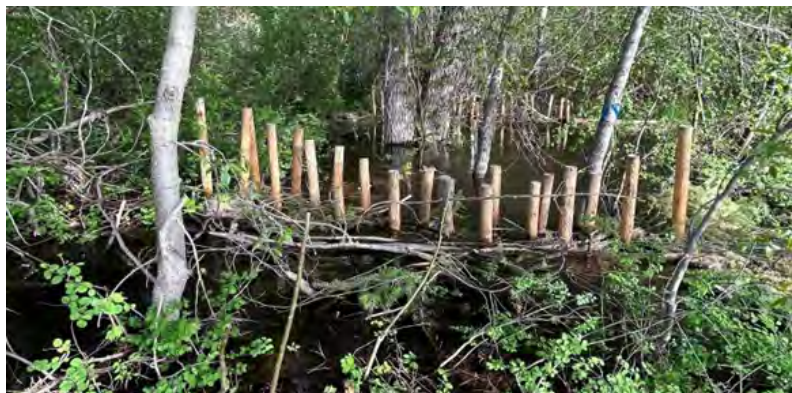
Figure 34: Methow Okanogan Beaver Project BDA installation showing beaver beginning to build upon the BDA that is located near a beaver relocation release site near Twisp, WA. Photo Credit: Jackie Corday.
